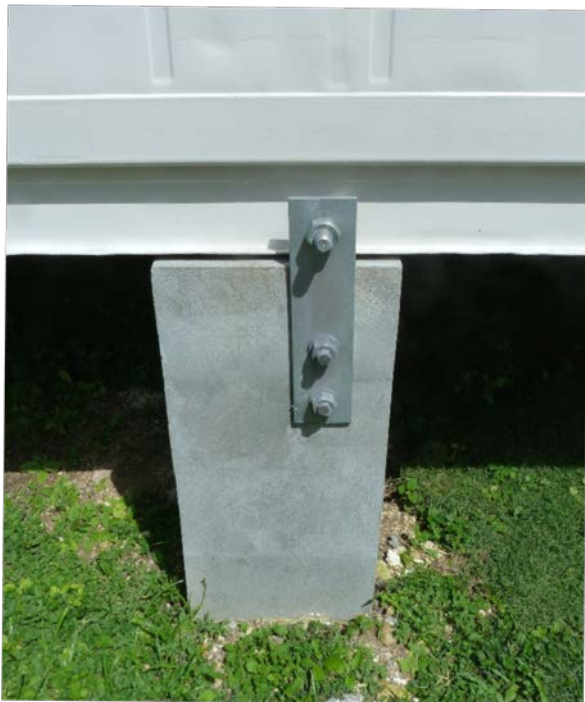
Figure 2. Current mobile rearing unit (MRU) anchoring system installation in Grand Cayman. End wall feature (A) and column feature (B).
